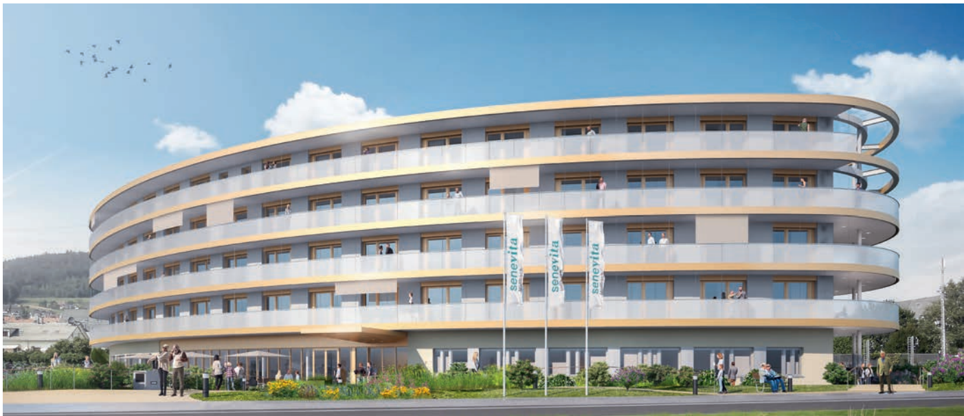
The Hycleen Automation System is suitable for new buildings such as the senior and care center Senevita Mülibach (Switzerland). Source: Senevita AG
